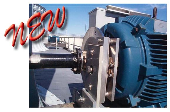
A simple mechanical brake for stopping, holding and locking out industrial fans, turbines, and other large rotating equipment
